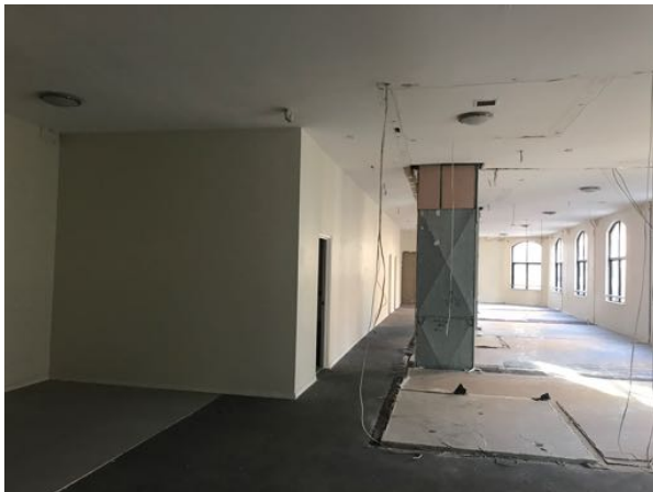
Figure 44: Nos. 761-763 George St First Floor interior.
