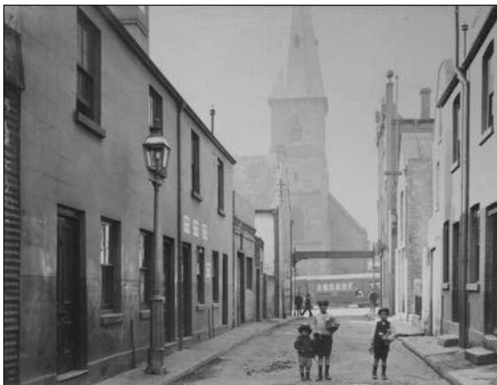
Figure 13: East facing view along Valentine Street prior to resumption and street widening in 1910 (NSCA CRS 51/2653).
