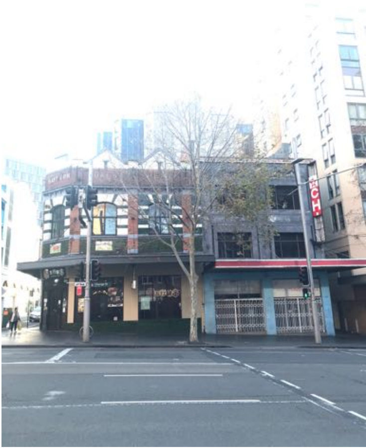
Figure 36: The site as viewed from George Street.
